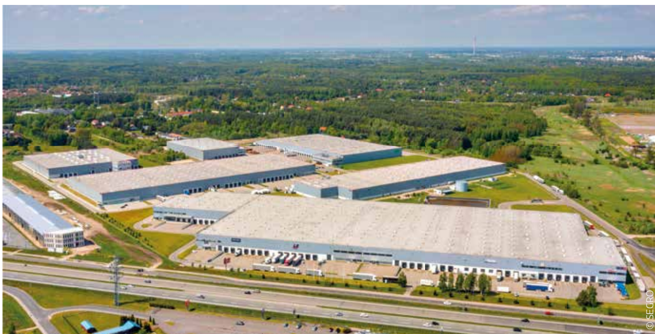
Fot. SEGRO Logistics Park Warsaw, Nadarzyn
